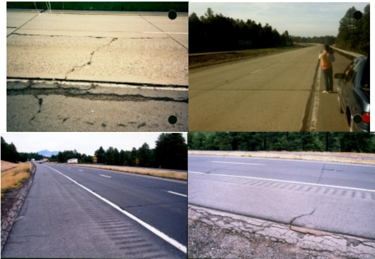
Figure 5. Before photos on top, after photos below
