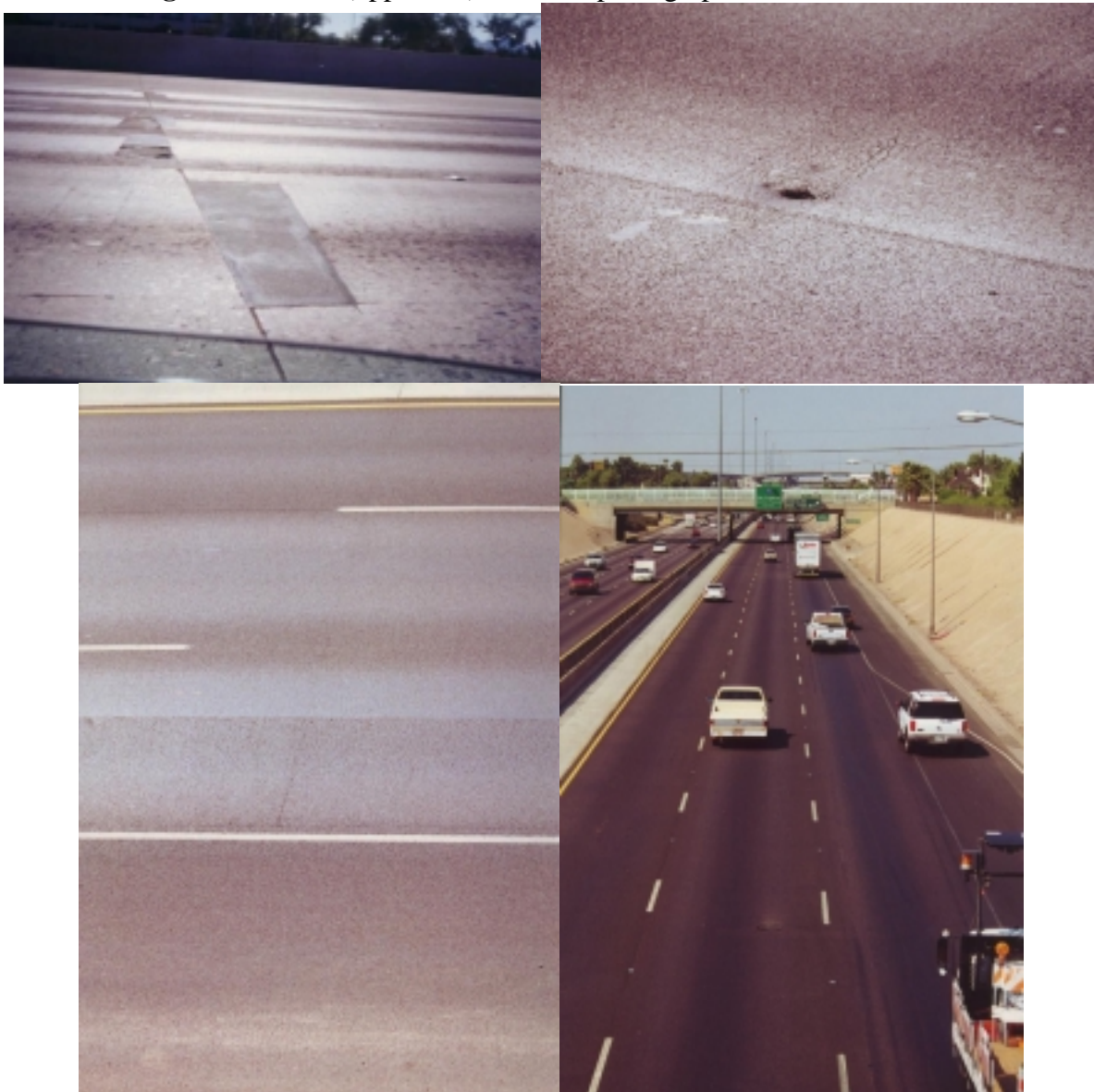
Figure 4. Before (upper left) and after photographs of I-17 in Phoenix
